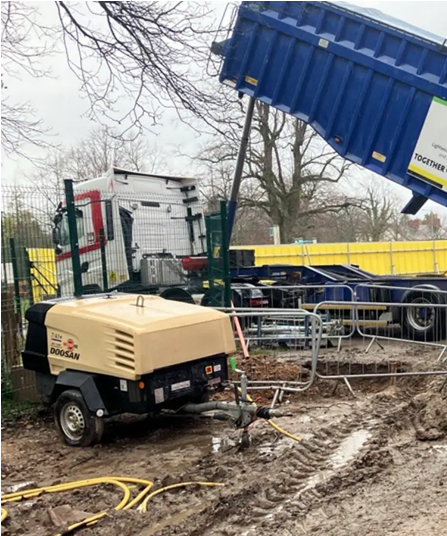
Lightweight Backfill Solution for Swimming Pool Construction
