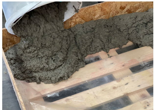
Step 4 40 Minutes Spread the material across the entire area to be filled
