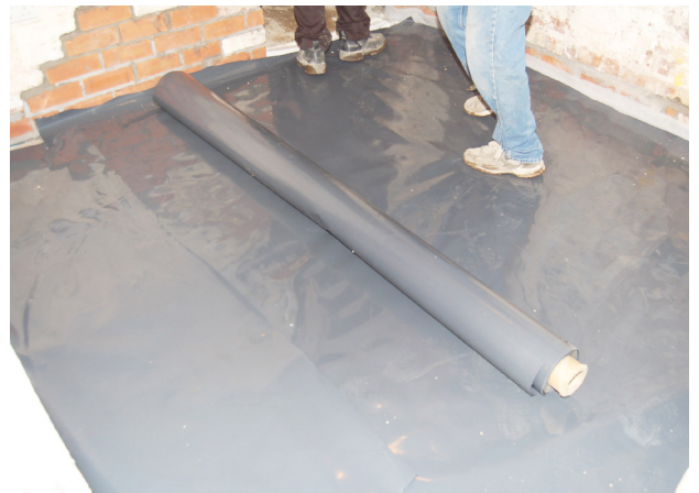
Step 4 40 Minutes Lay a 1200 gauge damp proof membrane
