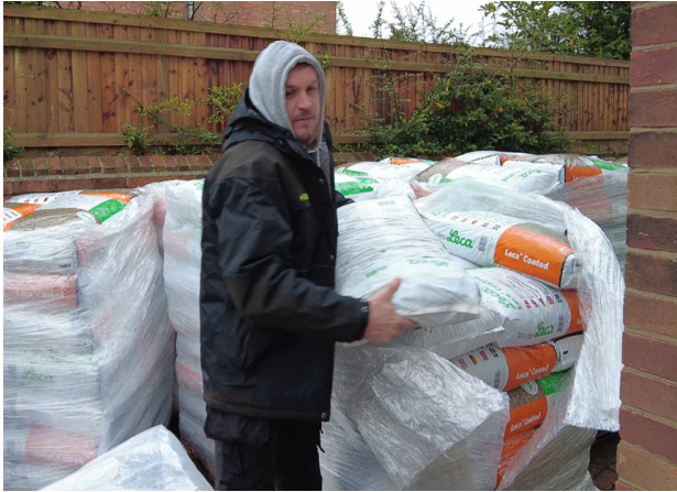
Step 1 10 Minutes Carry palletised bags into the property
