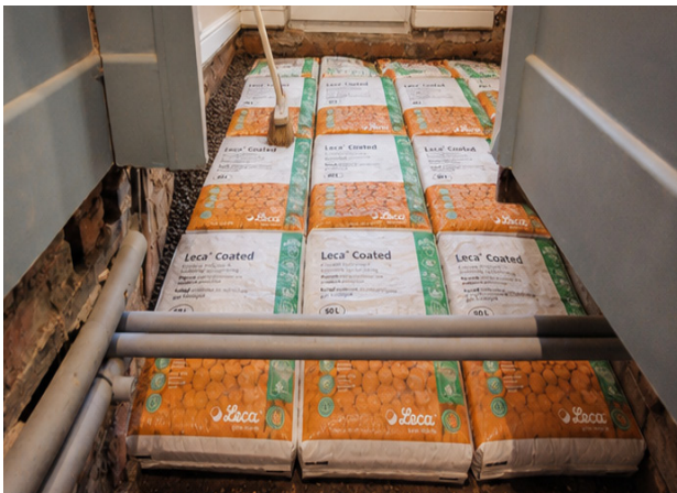
Step 3 30 Minutes Use loose material to fill any voids & level the surface
