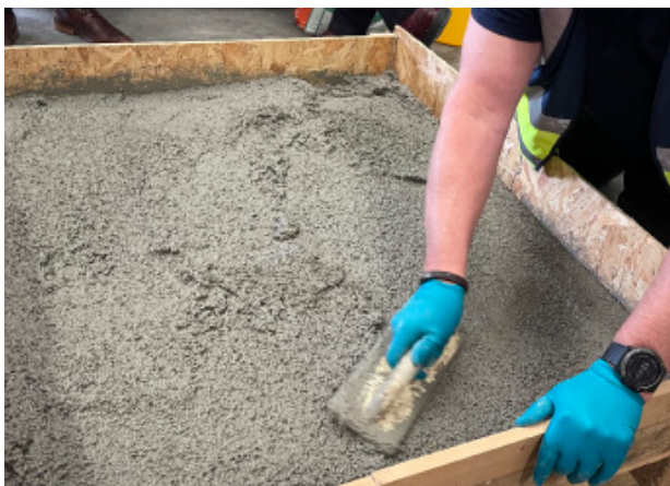
Step 5 60 Minutes Level to the desired thickness using a level and regularize with a manual or
