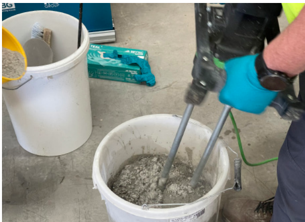
Step 3 30 Minutes Use a continuous mixer, the amount of water must be adjusted to the type
