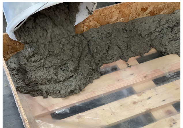
Step 4 40 Minutes Spread the material across the entire area to be filled
