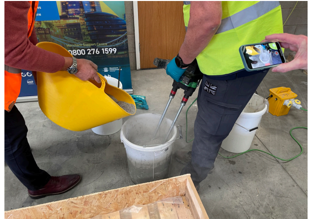
Step 2 20 Minutes Mix Leca Uno with water (5L/ per bag)
