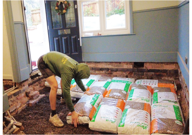
Step 2 20 Minutes Lay the bags on the ground
