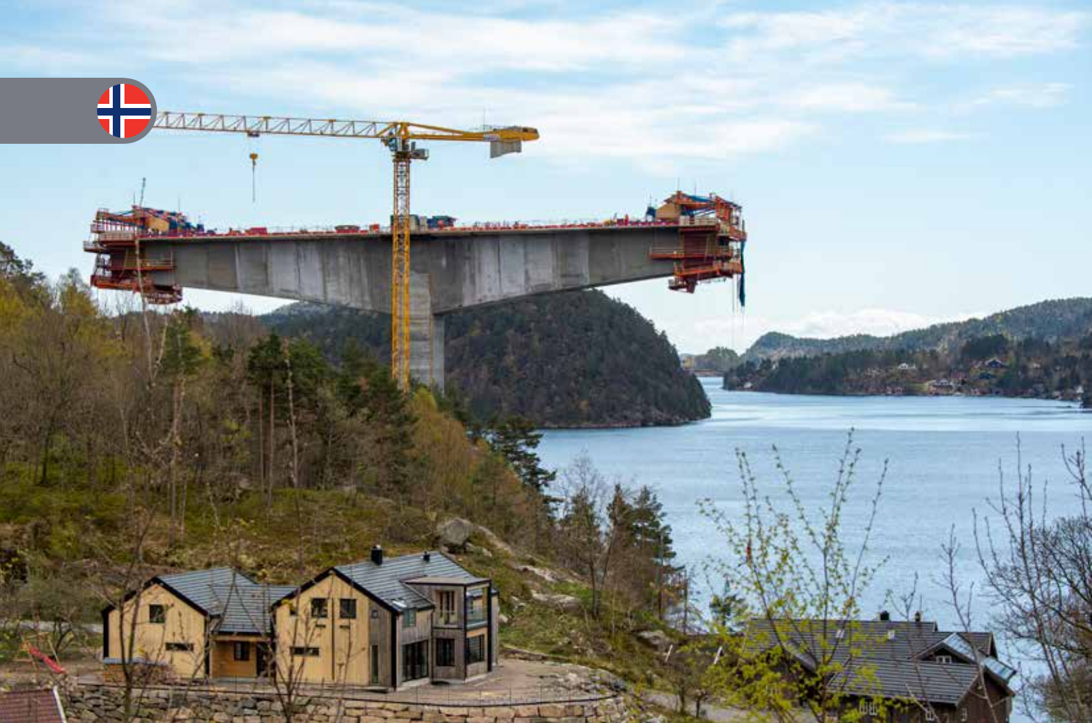
The casting of 260 meters long spans straight into the air, 64 meters above Trysfjorden, is right up to the limit of what is possible.
