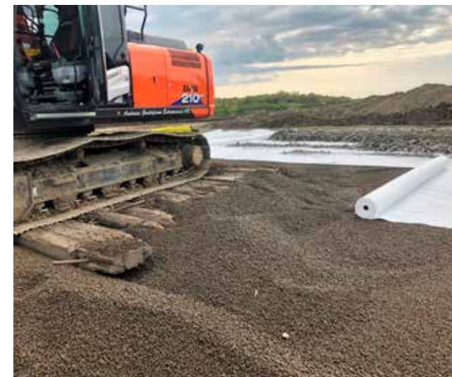
A layer of geotextile is first layed out before installing the Leca LWA.
