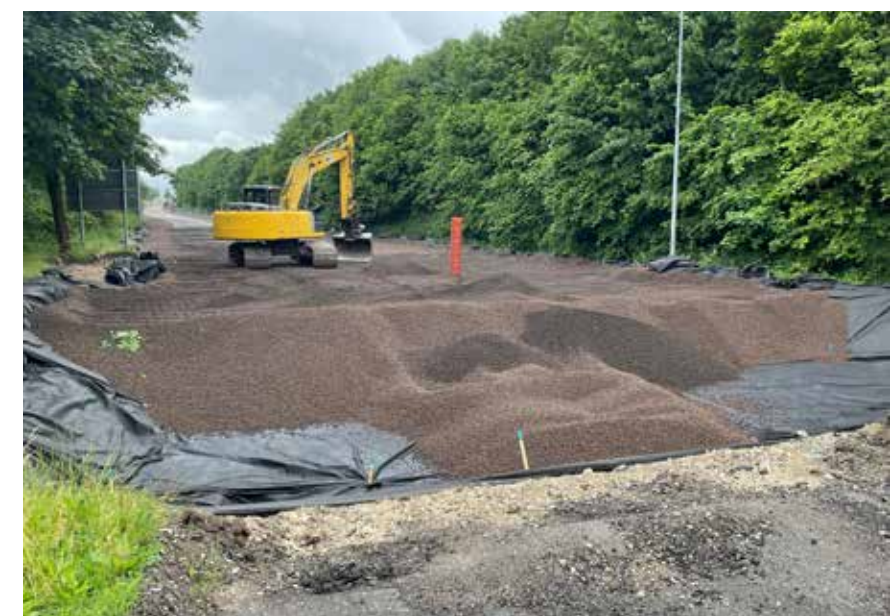
The LWA was laid in a 1 meter thick layer and compacted with crawler excavator.
