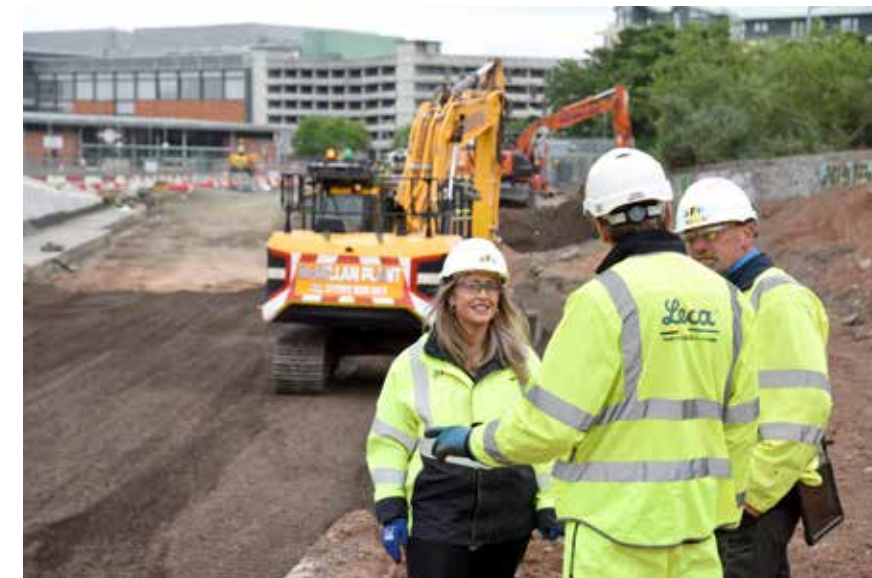
Leca LWA was specified as a lightweight solution to provide a robust foundation support for the track bed between two existing retaining walls
