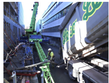
Cramped conditions on the construction site are no obstacle when the filler can be blown into place with long hoses (Photo: Jan Vestre)
