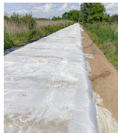
Structural fill in the form of “mattresses” made of lightweight expanded clay aggregate wrapped in geosynthetic fabric
