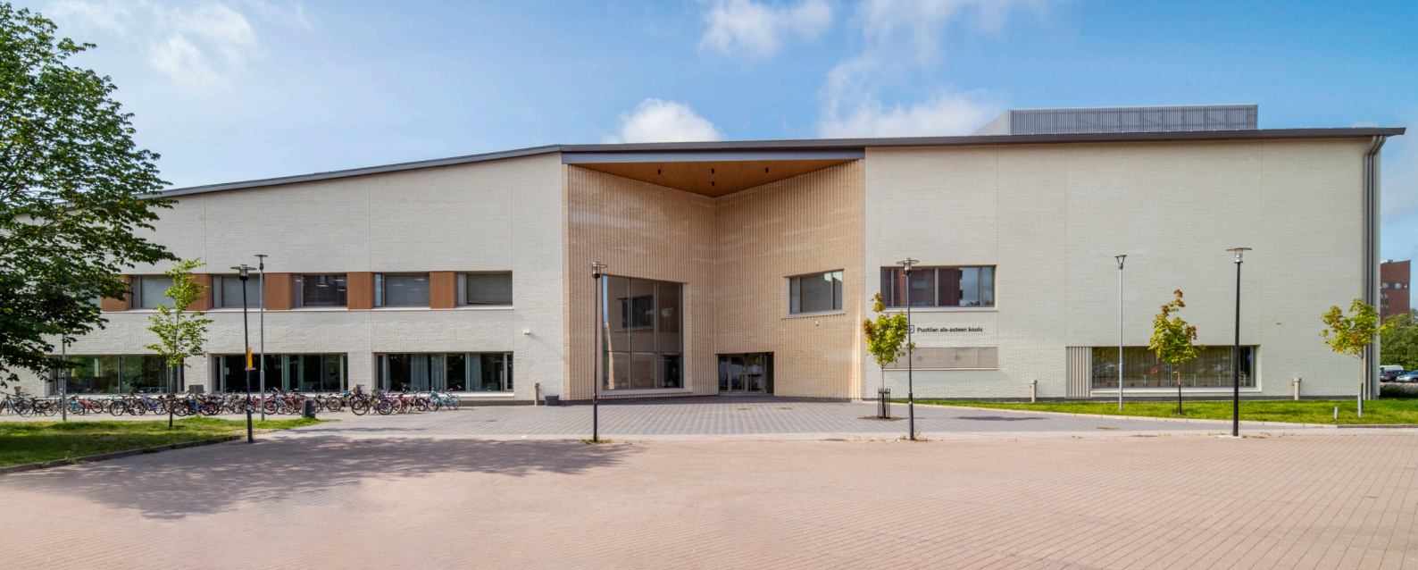
The newly built Puotila school provides a sustainable and spacious setting for students.
