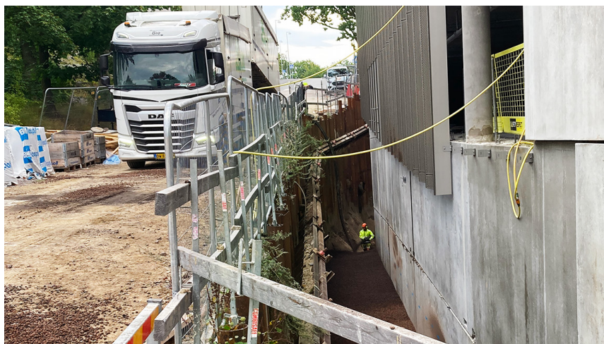
LWA is delivered by blowing to reach hard-to-access trenches at the parking structure.
