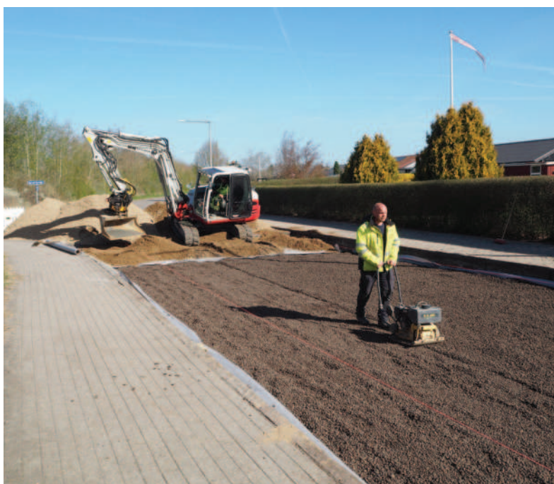
Leca LWA replaces sand as bottom protection
