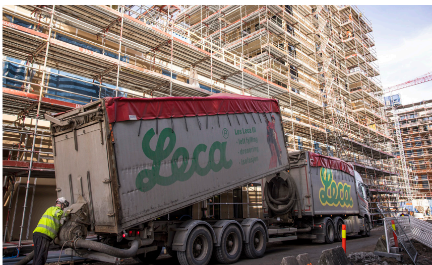
It is quick and easy to install Leca LWA compared to alternatives like polystyrene, which would require extensive use of construction cranes and more manpower.
