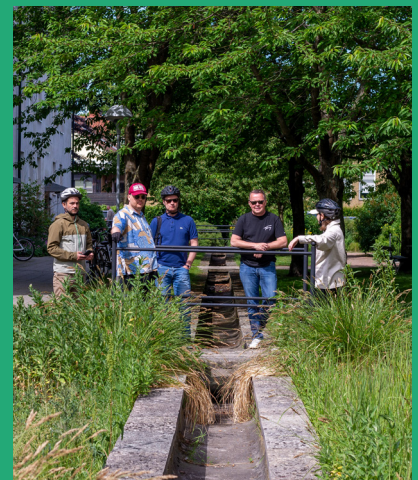
The channels in Augustenborg relieve pressure on old drainage systems by managing rainwater. Photo, Essi Malinen-Lallukka
