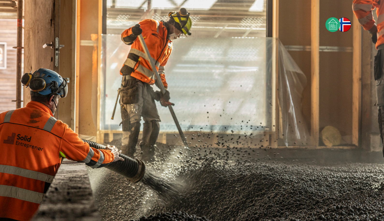
Leca LWA is blown into place directly from the truck, practically pre-compacted, with no need for manual unloading. It's hassle-free to walk on and requires zero packaging.
