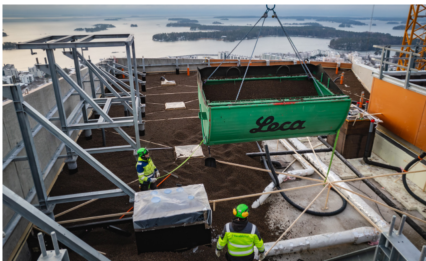
Skilled workers from Kerabit Katto Oy expertly handle the Leca LWA installation.
