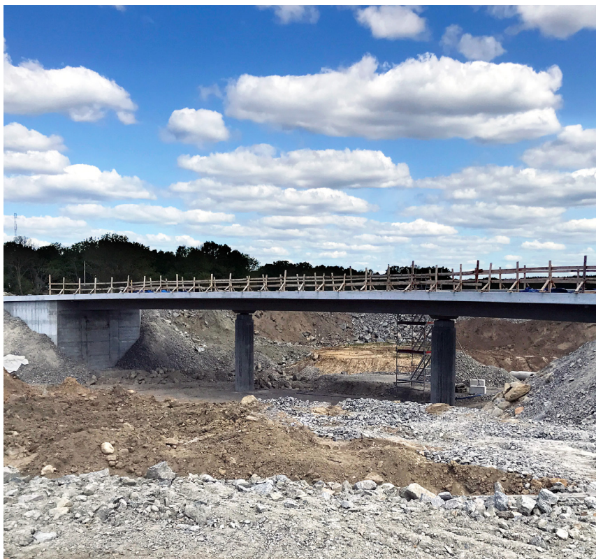
One of the 23 bridges being built to enhance infrastructure, where Leca LWA prevents additional piling.
