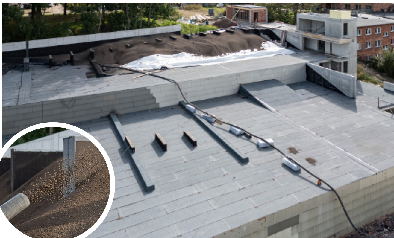
Leca LWA was pneumatically delivered directly onto the roof structure.
