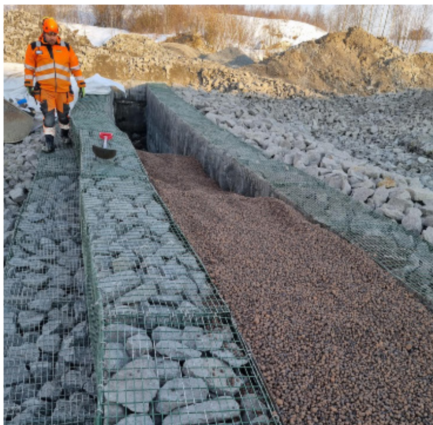
Leca LWA placed in the dam core, easy to replace.
