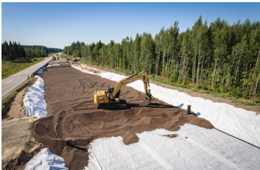
Leca LWA layer 1.3–3.3 m, enclosed in geotextile.
