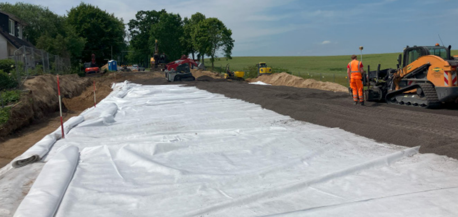
Leca LWA was enclosed in a geotextile
