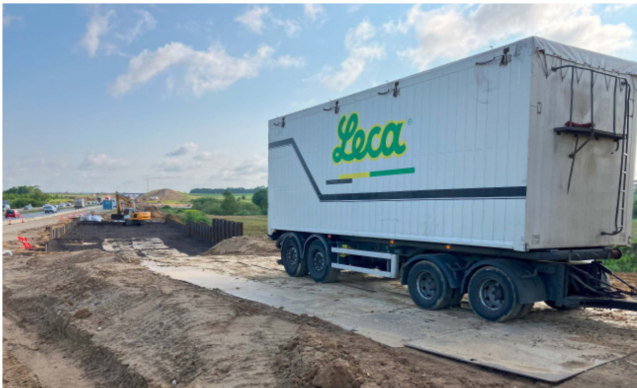
Delivery of Leca® lightweight aggregate for the E45 expansion. The material arrives ready for placement, ensuring an efficient construction process.
