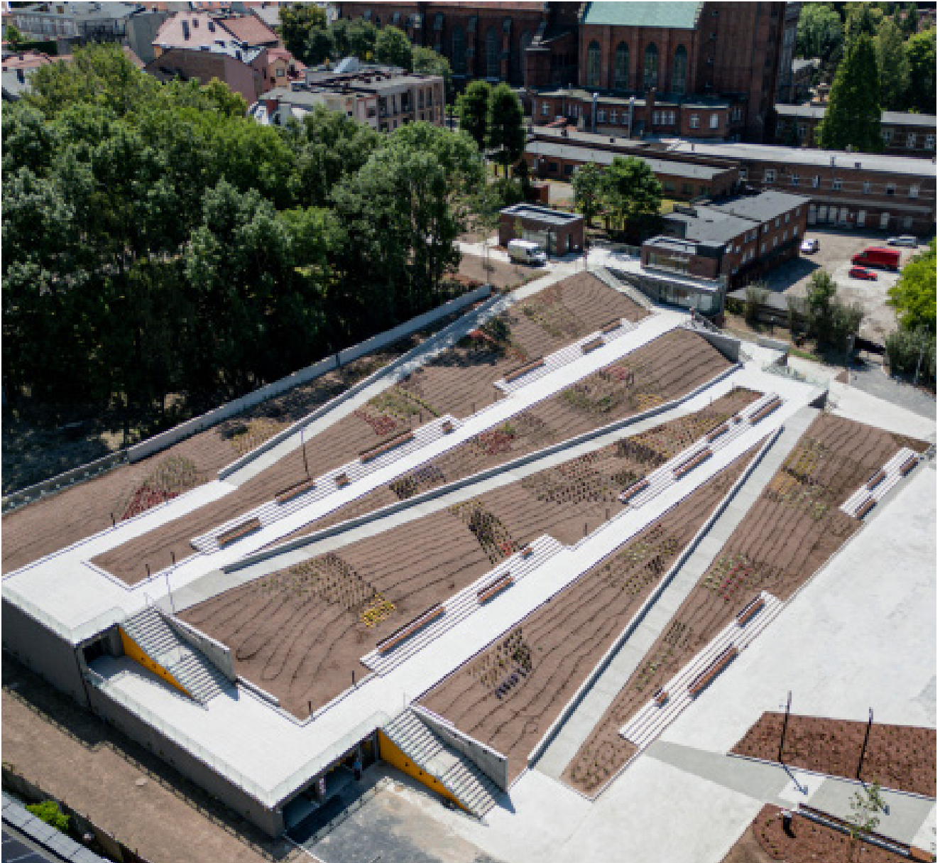
Leca LWA was selected for its reduced weight, minimal water absorption and excellent drainage capacity
