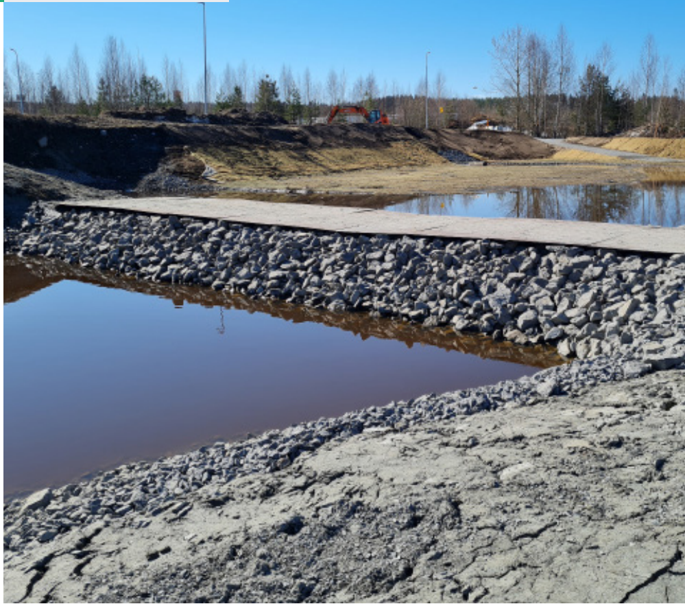
Completed dam filters water before discharge.
