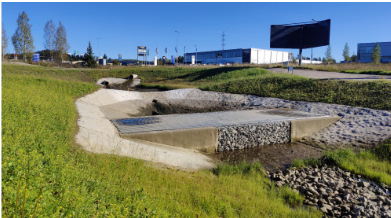
In Nikkilä, the filter dam completes treatment.
