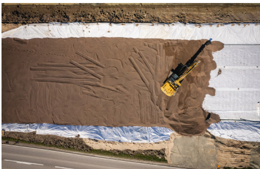
Leca LWA was compacted with a crawler excavator.
