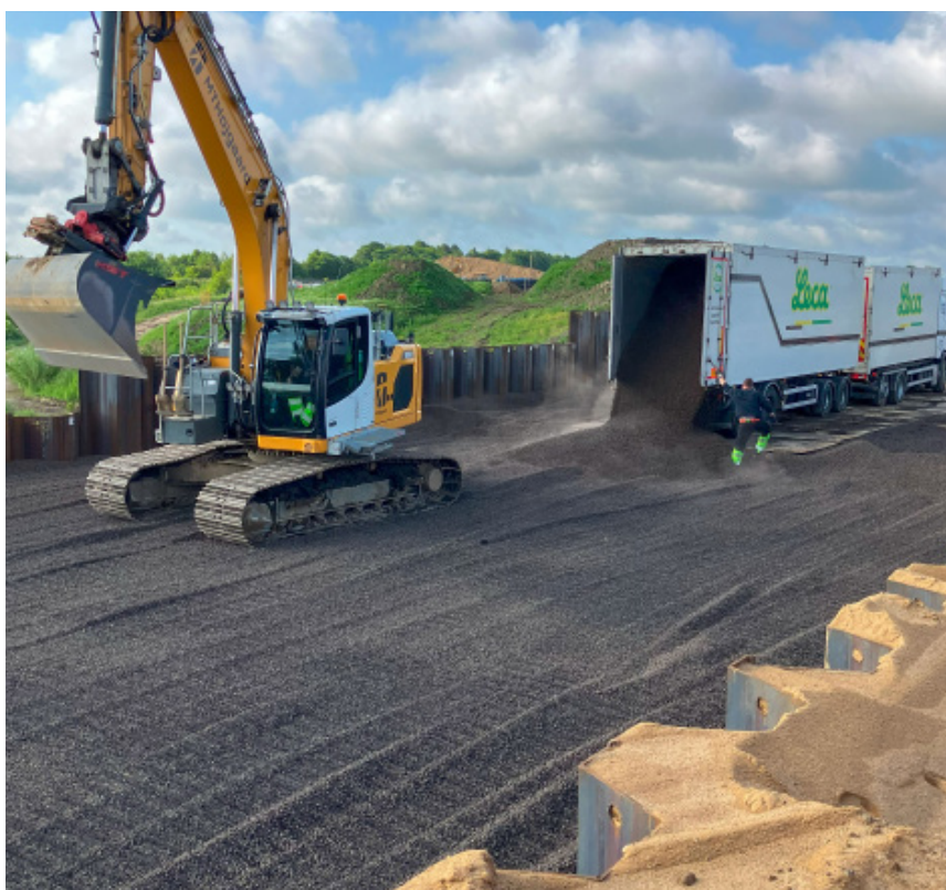
Leca® lightweight aggregate being placed on the E45 motorway — reducing load and earth pressure in the road structure.
