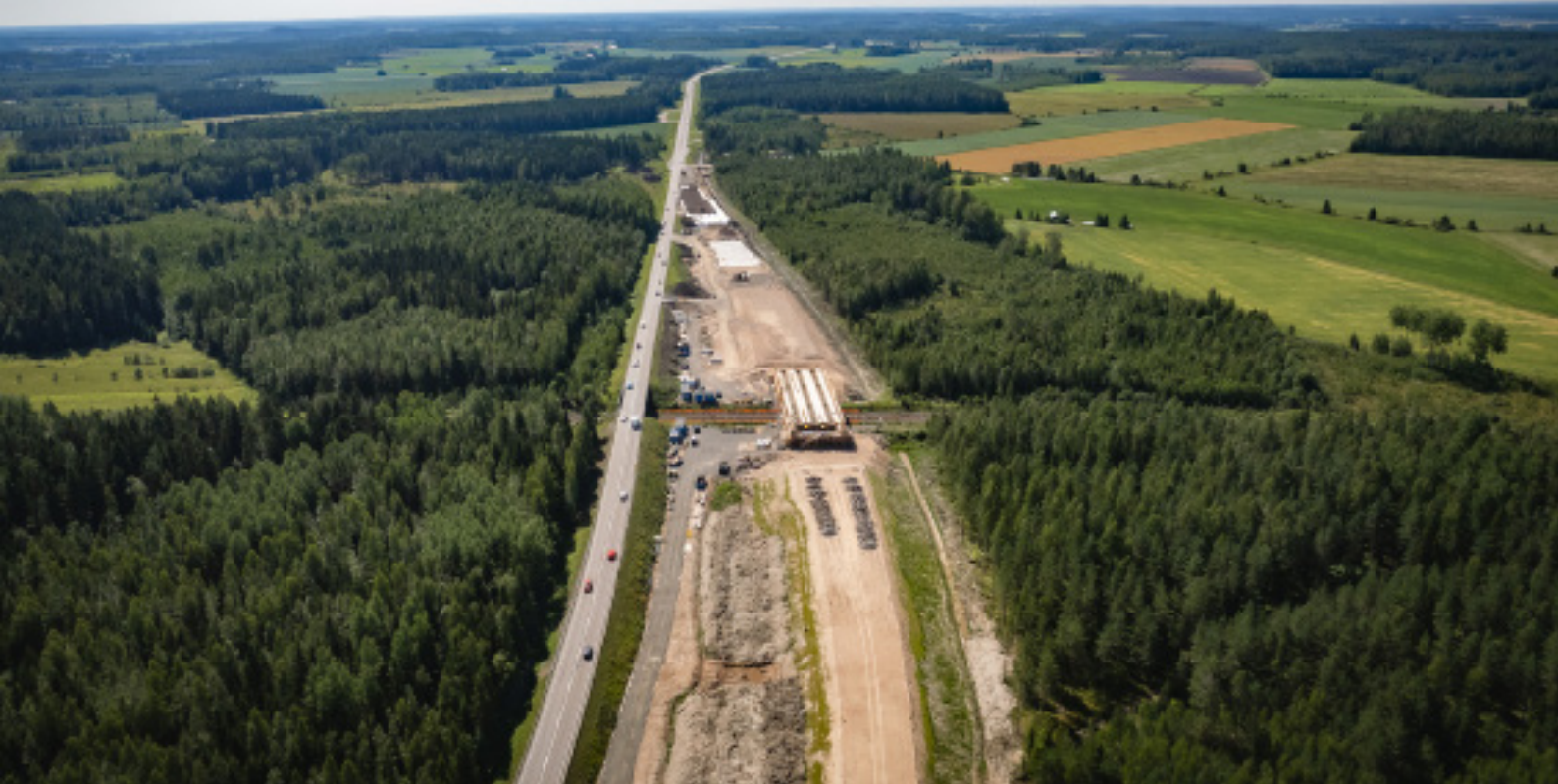
Aerial view of the construction site at Korja.
