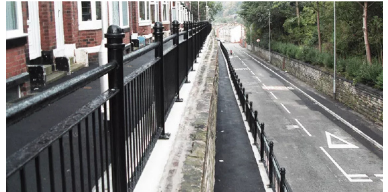
The existing wall was over 100 years old
