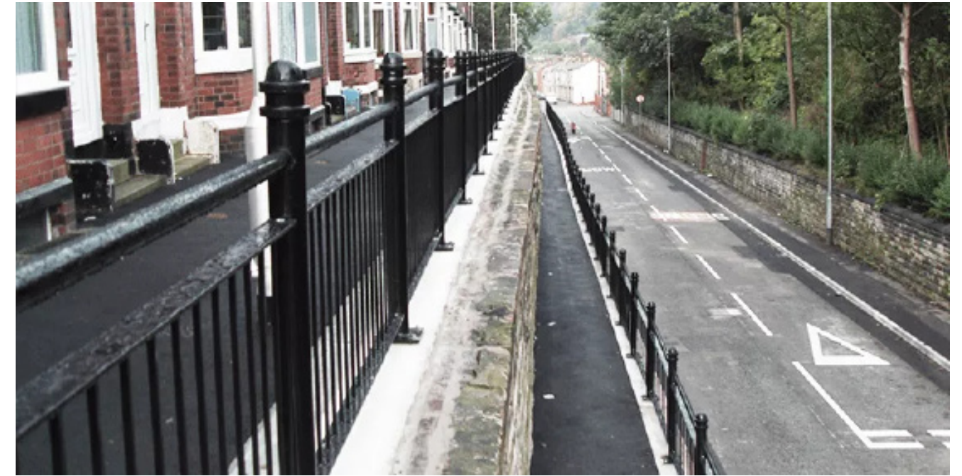
The existing wall was over 100 years old
