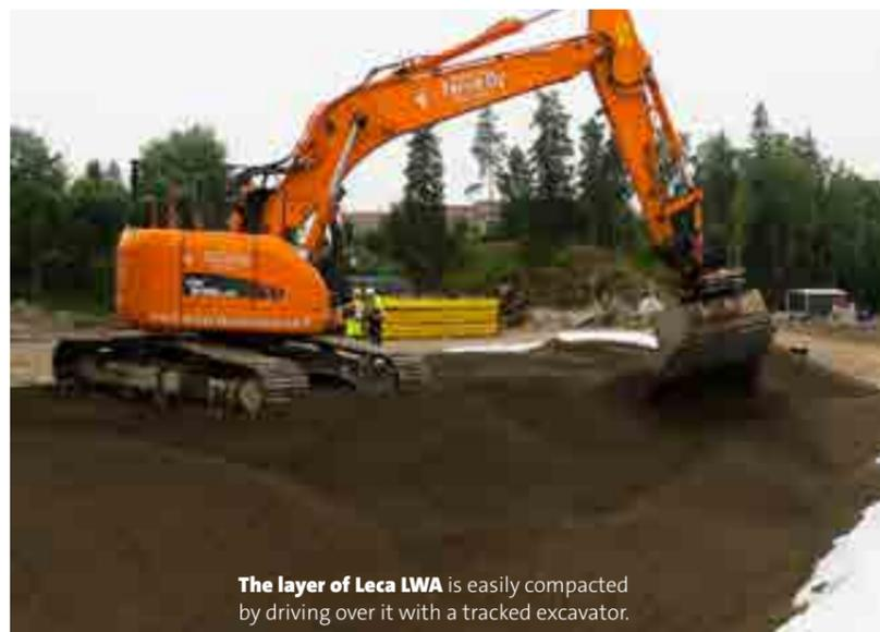
The layer of Leca LWA is easily compacted by driving over it with a tracked excavator.
