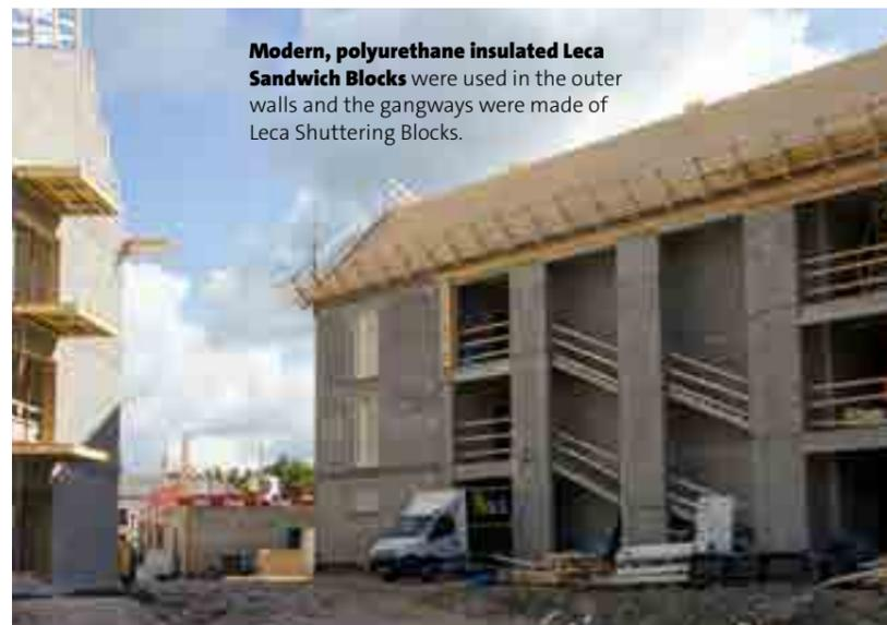
Modern, polyurethane insulated Leca Sandwich Blocks were used in the outer walls and the gangways were made of Leca Shuttering Blocks.
