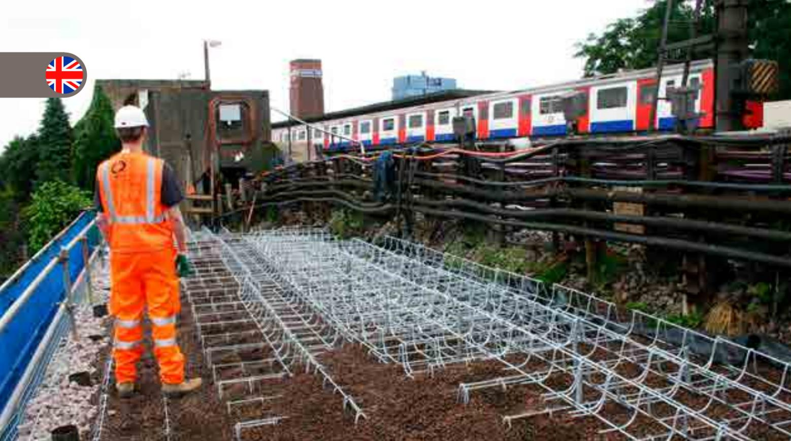
As a **Lightweight Backfill** the Leca LWA was placed within the Ramwall system
