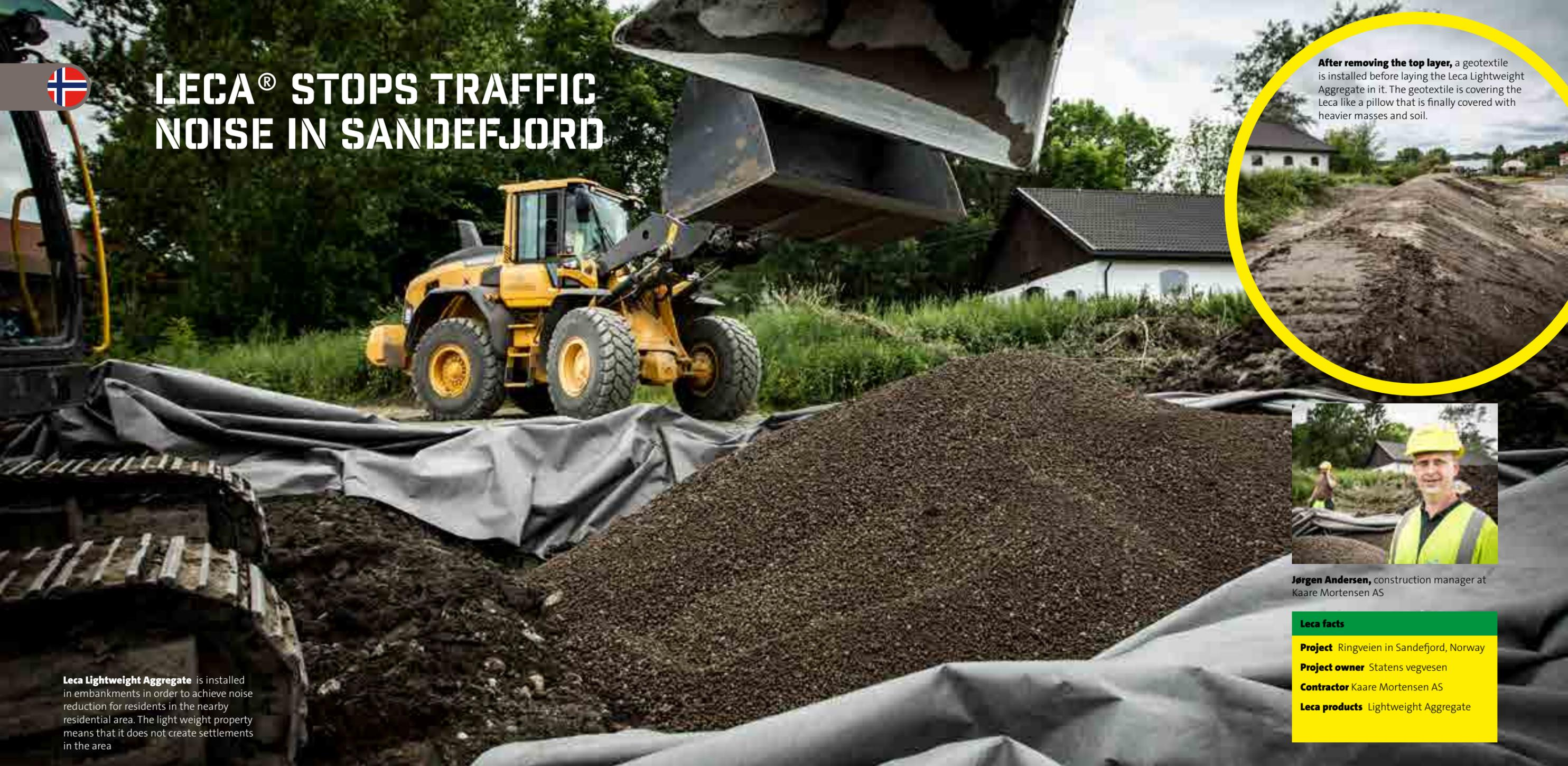
After removing the top layer, a geotextile is installed before laying the Leca Lightweight Aggregate in it. The geotextile is covering the Leca like a pillow that is finally covered with heavier masses and soil.
