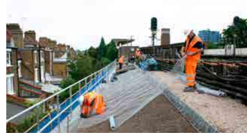
Stabilizing the embankment walls along a 200 meter stretch of the Acton Town to Chiswick Park for the London Underground.
