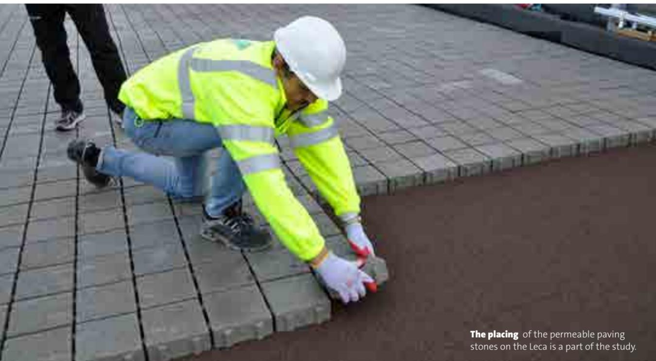
**The placing** of the permeable paving stones on the Leca is a part of the study.
