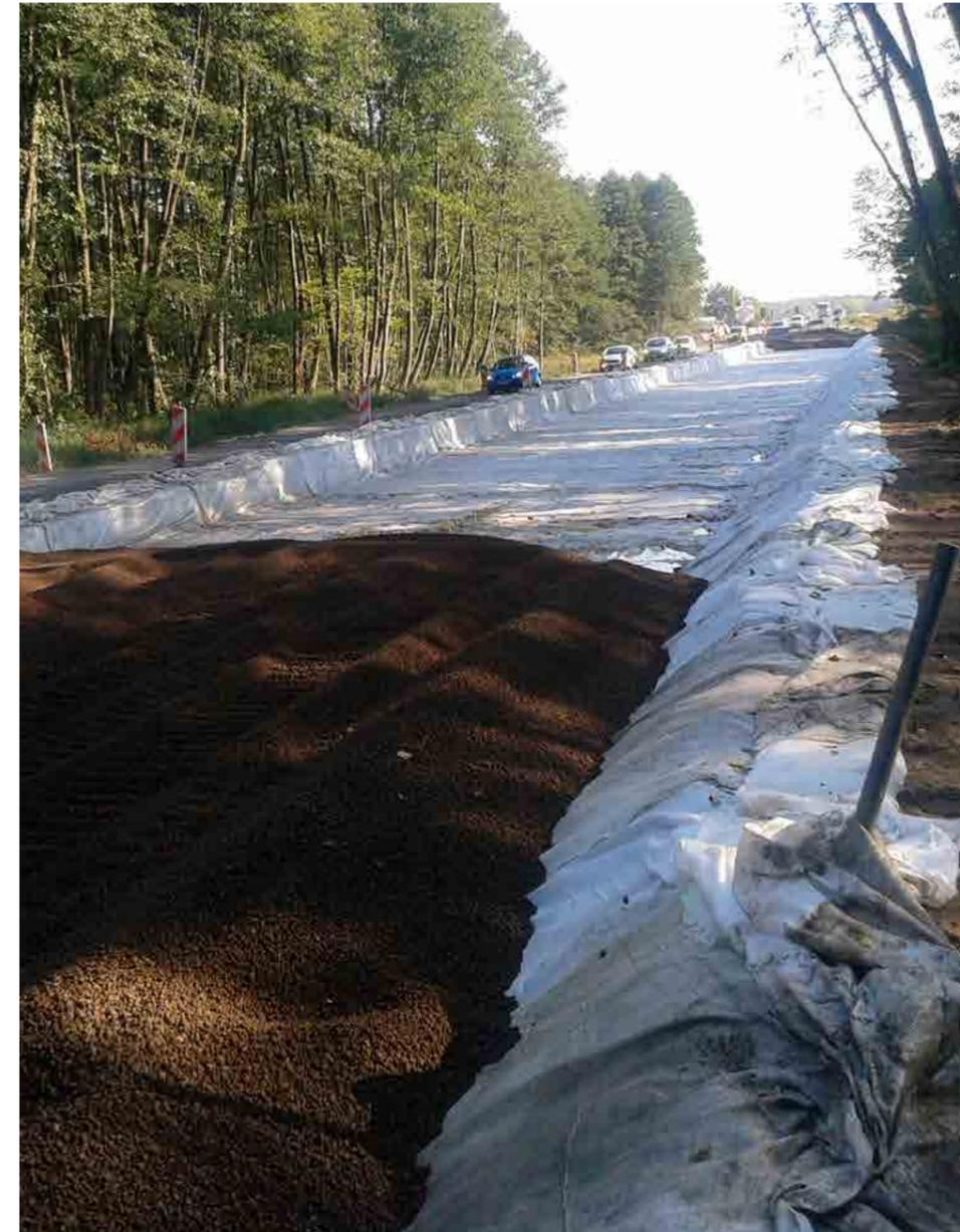
aggregate that was wrapped with a polyester geotextile, and a reinforced embankment construction (0/63 mm crushed-stone aggregate + polyvinyl alcohol geonet).
