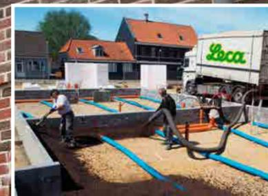
The Leca® LWA was delivered by our smart blowing truck for an easy installation.
