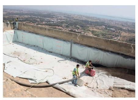
Leca LWA was pumped directly through pneumatic delivery.
