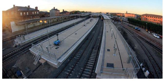
lightweight solution for the rail platform. The lightweight fill was used behind the riser walls in order to reduce loads applied. Leca LWA was specified in areas where small foundations were installed to accommodate electrical cabinets on the platforms. The cabinets were installed on top of the Leca LWA.
