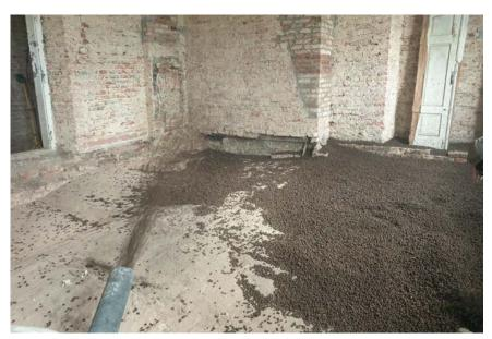
Aggregate laying with the use of a pump.
