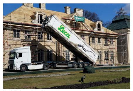
Vehicle with a pump for feeding aggregate.
