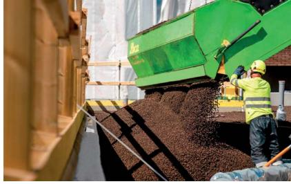
Leca LWA was delivered quickly and easily with a lifting box.
