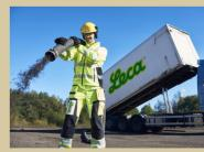
2. **Pneumatic Delivery** - Leca® LWA benefits from its ability to be pneumatically delivered. The LWA is blown out through a 5 "hose at a rate of 1 m3 per minute.
