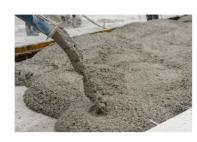
Leca® Lightweight Aggregate Concrete (4-10mm) is mainly used as an additive in industrially manufactured Concrete. One of the primary benefits of using Leca® Lightweight Aggregate Concrete in lightweight concrete production is its reduced density.
