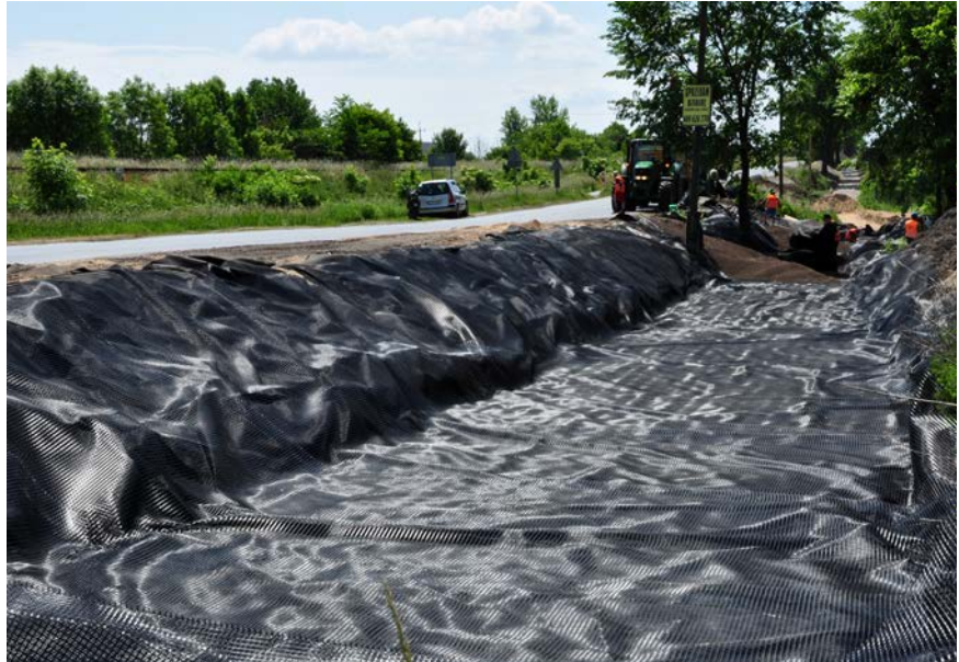
Geotextile layering
