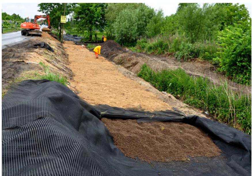
Covering the filling and sub-base for the pavement
