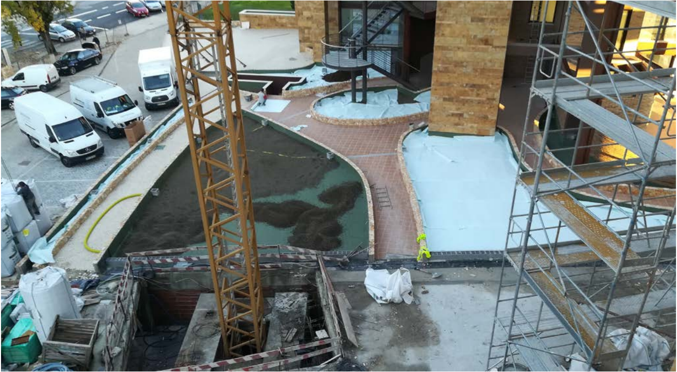
A total of 400 m 3 of Leca LWA, delivered in small and bulk bags, was used in this project.
