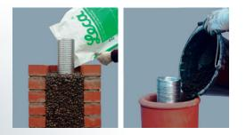
Fill with Leca<sup>®</sup> to just below top of the chimney prior to fitting capping or cowl.
