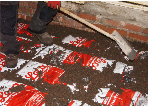
Step 3 30 Minutes Use loose material to fill any voids & level the surface
