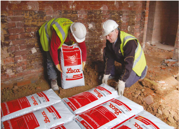
Step 1 10 Minutes Lay loose fill to level up the site
