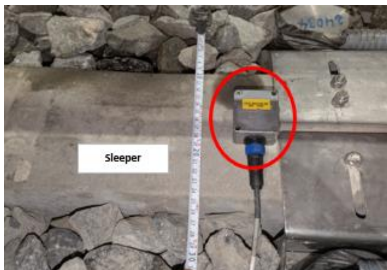
Figure 56.-Example of accelerometer located at sleeper
