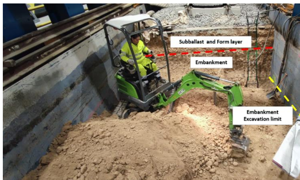
Figure 22.- Excavation of the embankment using machinery
