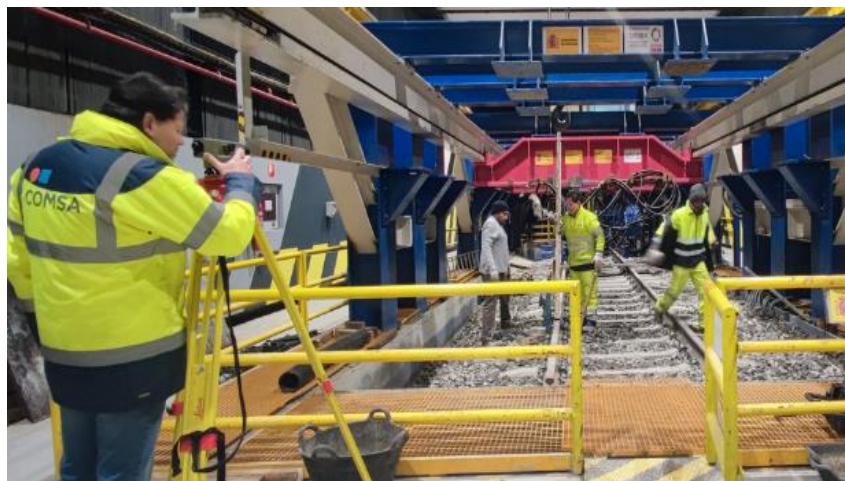
Figure 44.- Levelling of railway track sections.
