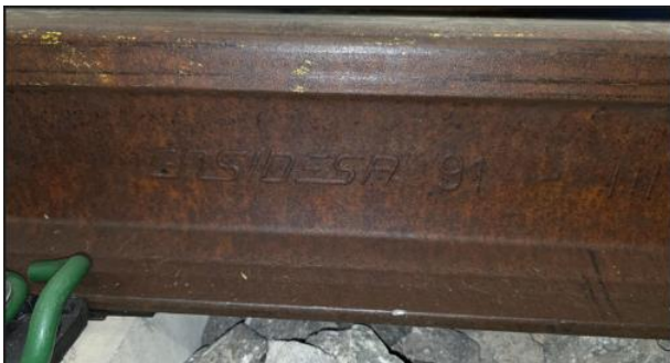
Figure 17: UIC 60 rail used in railway track section
