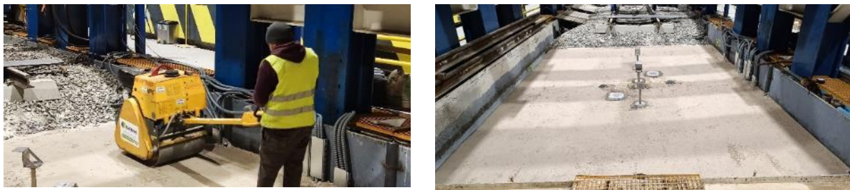
Figure 40.- Sub-ballast layer; left: new compaction machine, right: final aspect of sub-ballast layer
