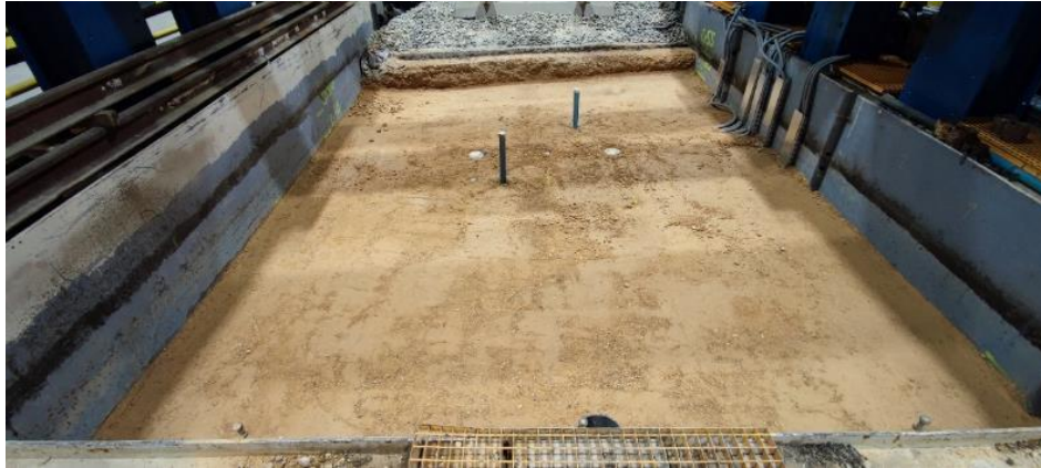
Figure 36.- Top of the form layer after construction
